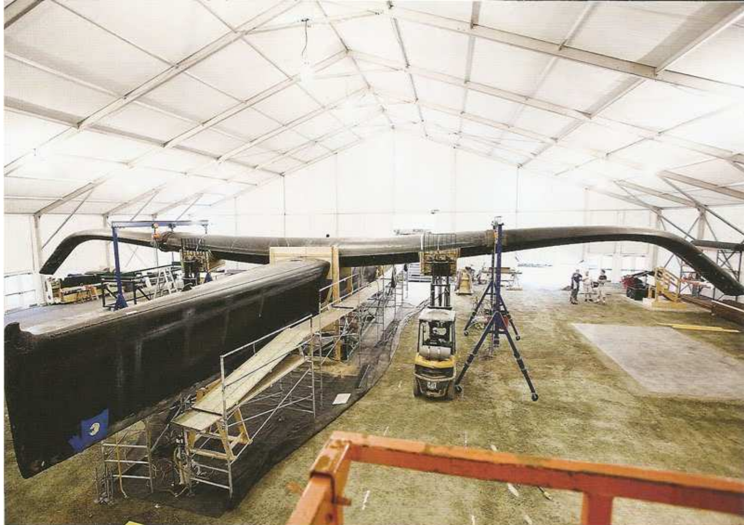
The main hull nears completion in Anacortes with the primary structural beam elements as the floats and remaining beam fairings are worked on 25 miles away. Without the benefit of an established multihull yard improvisation became a key theme throughout the build
