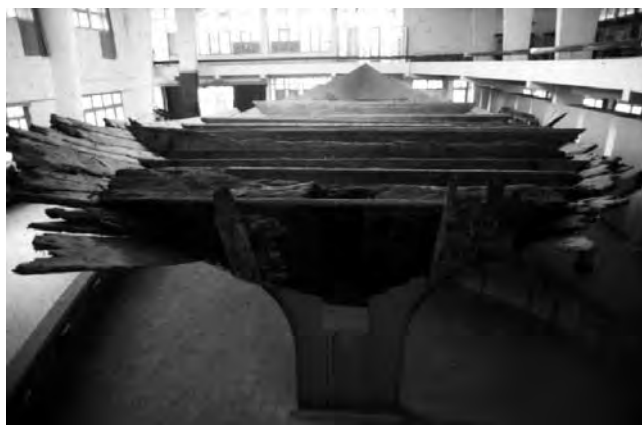
Figure 95. View of stern of vessel showing axial rudder slot.
