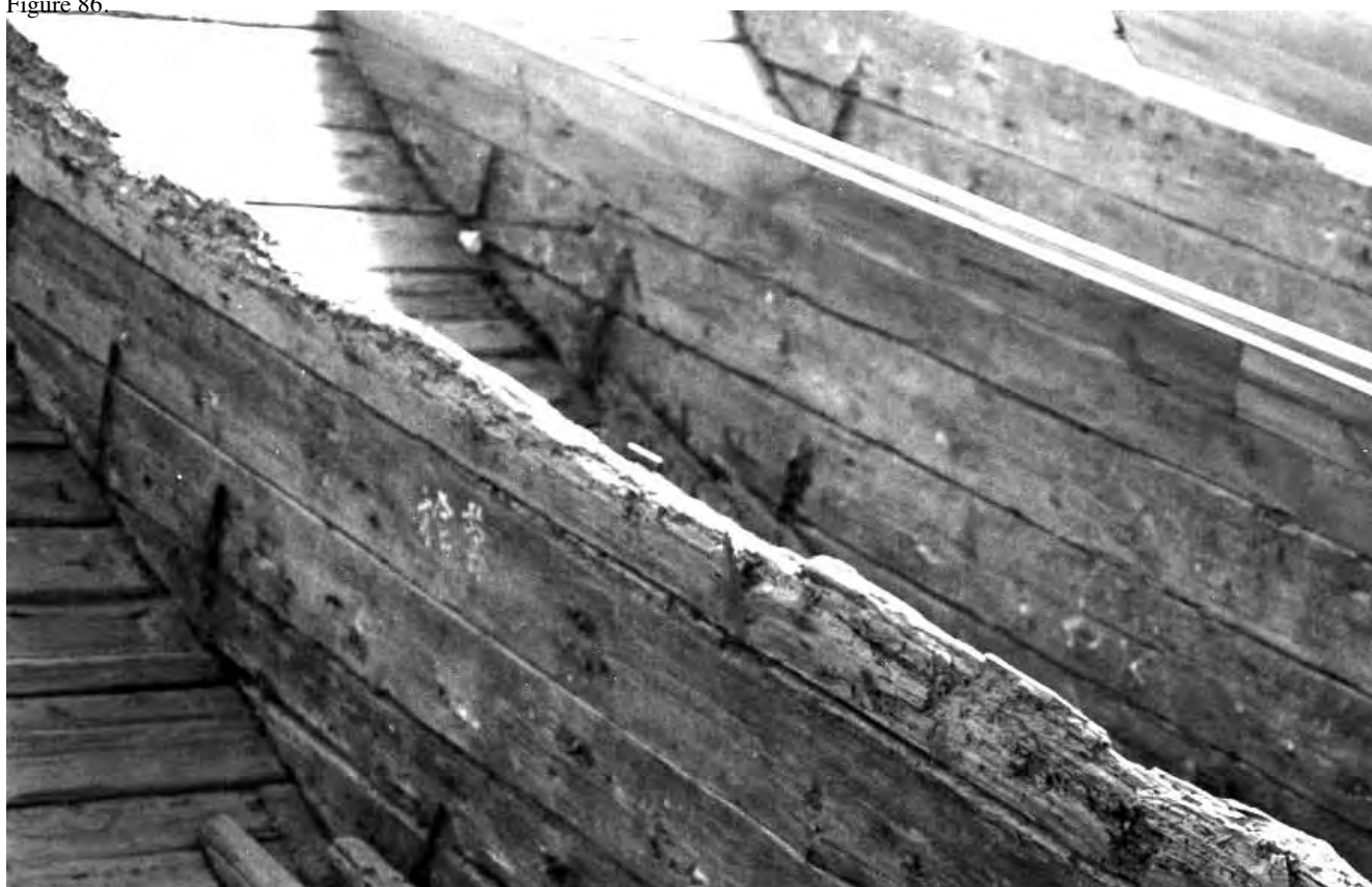
Figure 87. Bulkheads 7 to 10 (right to left).
